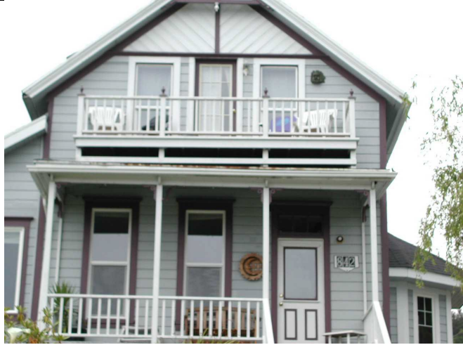
Correct: Support posts line up with 1 st and 2 nd floor; balusters are within proportions and meet historic characteristics.
